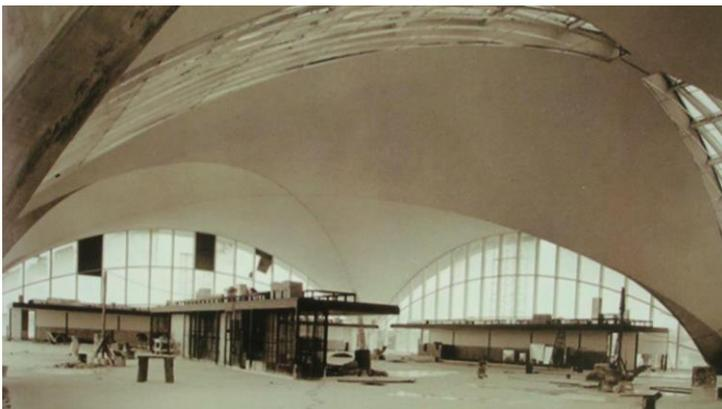
**THE JET AND SPACE AGE** - In 1956, Minoru Yamasaki's iconic arched terminal opened, becoming the forerunner of many modern airline terminals. Its modular design provided for later expansion. The first McDonnell
