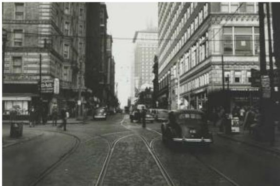
**TRACKS TO NOWHERE** - Another photo of disused streetcar tracks on 9th St at Pine looking North. The double track on 9th south of Pine was formerly used by the 73 Bellefontaine which was bussed in July 1947. The single track on 9th, north of Pine still has trolley wire to Olive where it could have been used as an emergency turnback. The single track on 9th north of Pine was last used by the 73 Bellefontaine line northbound.
