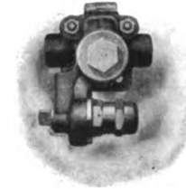
Fig. 501—Single-Pressure Feed Valve, Type C-6
